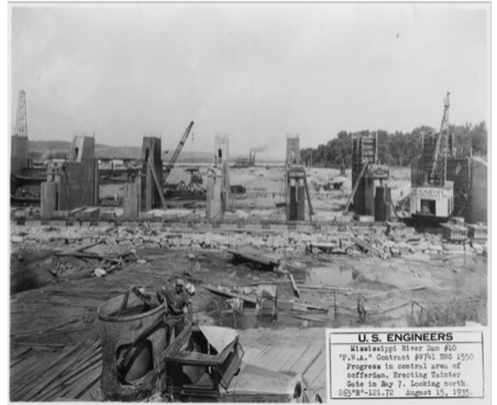
PWA Project and Army Corps of Engineers Lock & Dam #10 construction.
