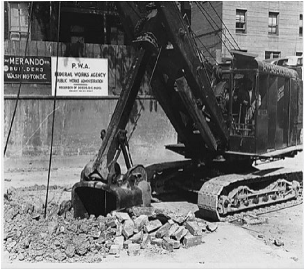
PWA-funded construction site in Washington, D.C. in 1933
